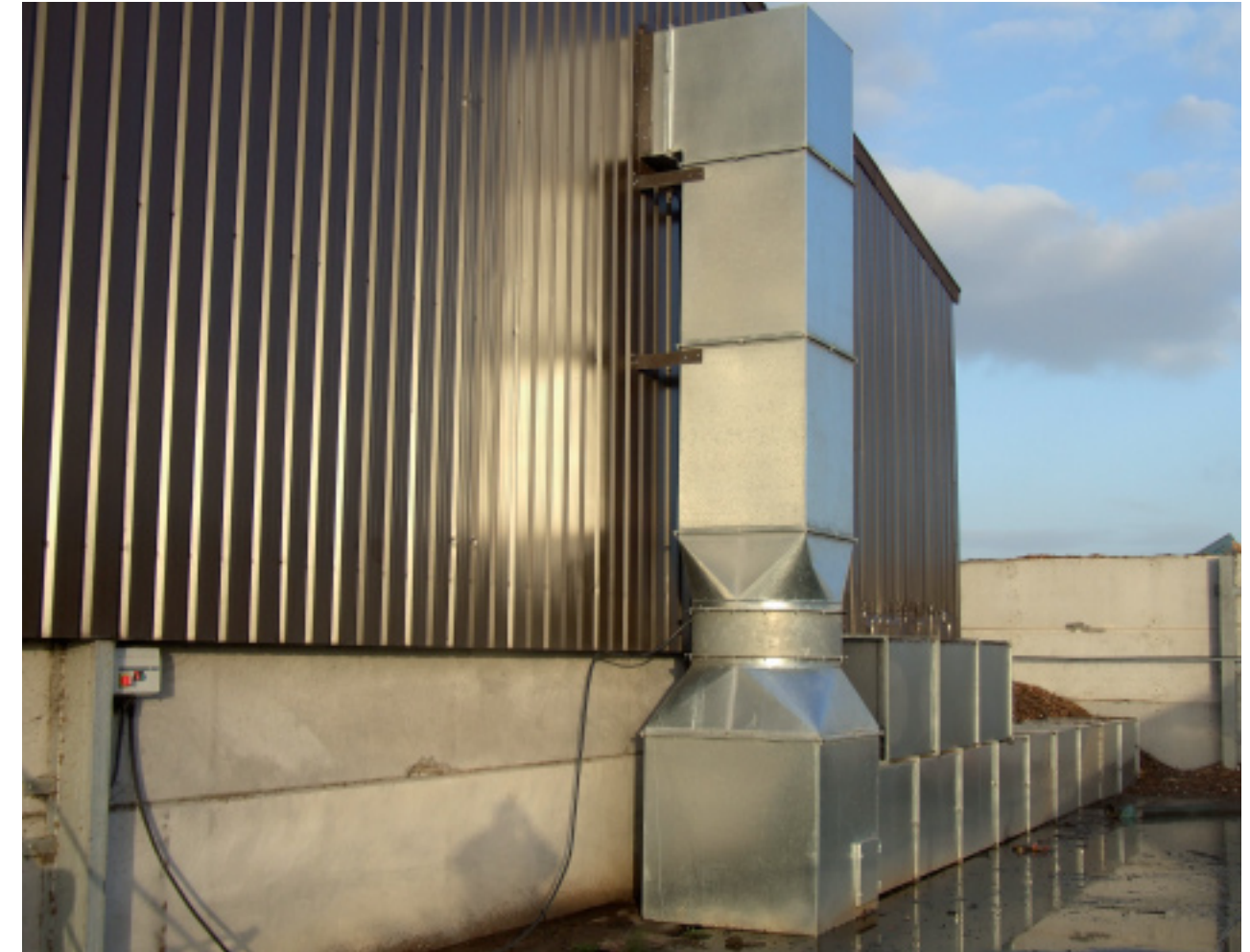
Figure 5 Illustration showing ductwork configuration at a biofilter in Dorset
