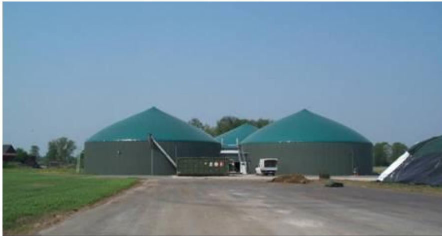
Photo 1: Anaerobic digestion plant in Germany
