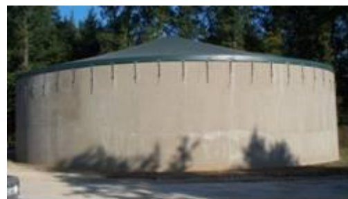
Photo 6: Covered digestate storage tank
